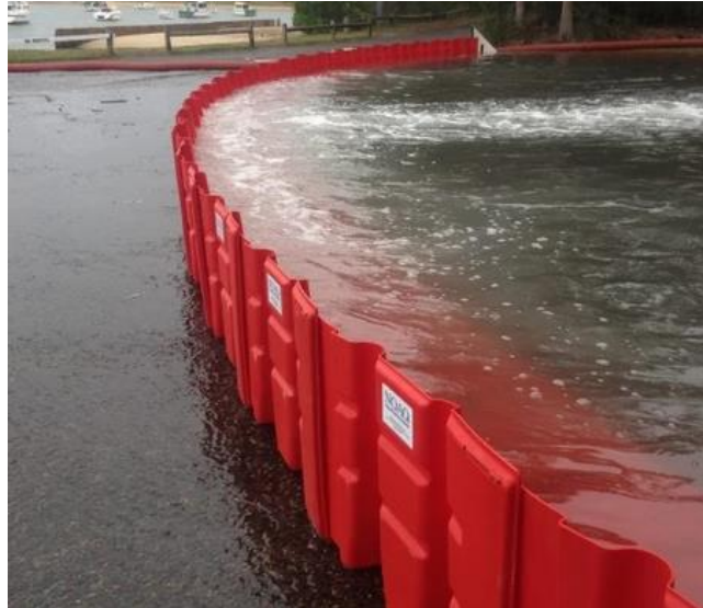
Figure 3. Plastic self-standing assembly elements
