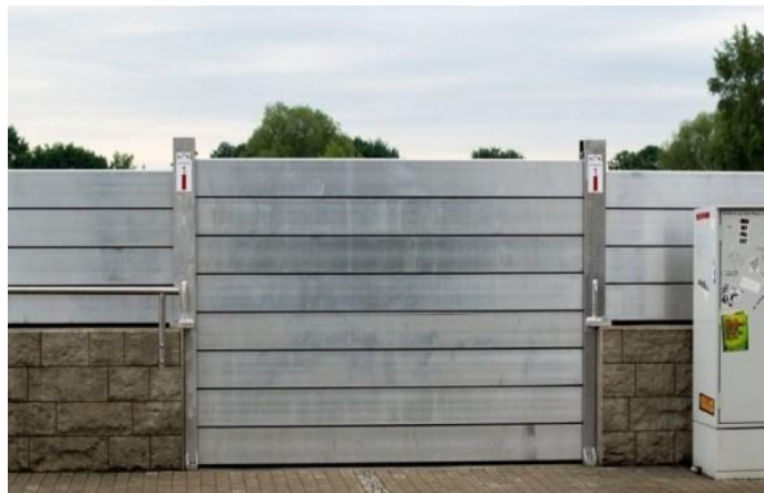
Figure 4. Pre-assembled metal panels
